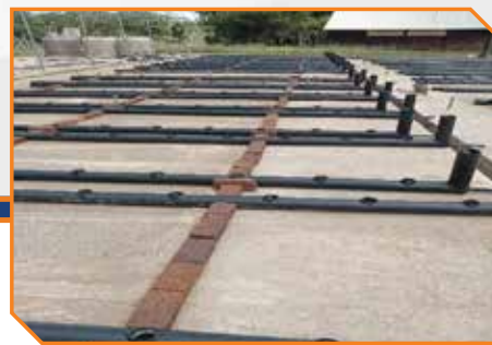
Pipes and syphon structure
