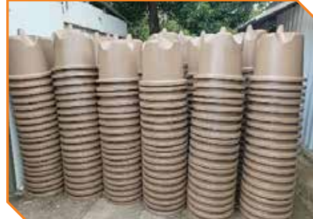
Gravel barrels in place and ready for pipes and syphon structure installation onto the pipe and syphon structures
