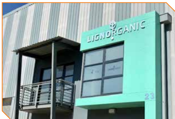
Figure 32: The LignOrganic facility
