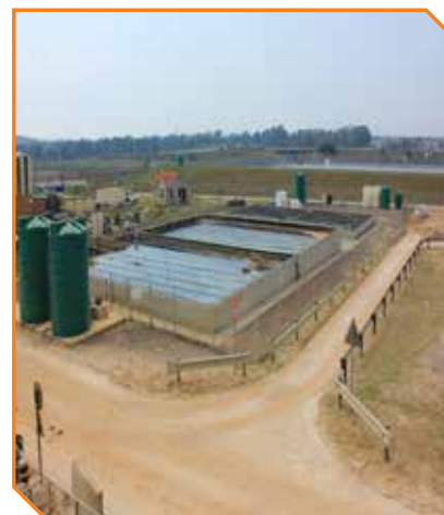
Figure 21: View of the cloSURE™ system at Thungela
