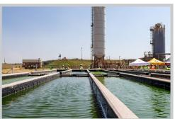
The technology is a semi-passive biological process for the treatment of mine impacted waters after mine closure, to produce water fit for re-use, specifically in agriculture. It is based on bacteria that act on sulphates which are common in AMD.
