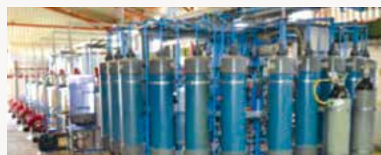
Figure 16: A ring of PLC-controlled multiport valves for resin regeneration; dilute nitric acid to regenerate the cation resin and methanol for the anion resin with a portion of the annex line at the back
